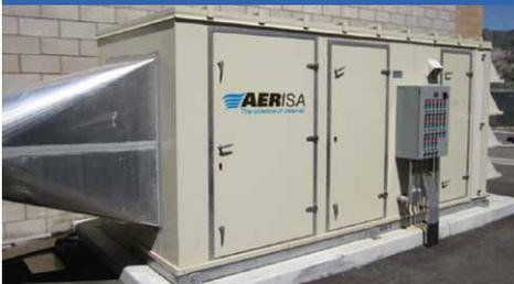
AerSupply with Ionizer Section
