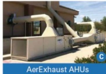
The Aerisa solution starts with generating positive and negatively charged ions in a supply air handler, which are then sent through a duct system into the facility to attack contaminants at their source. In most cases, the building air is ionized again in an exhaust air handler as it exits the facility.
