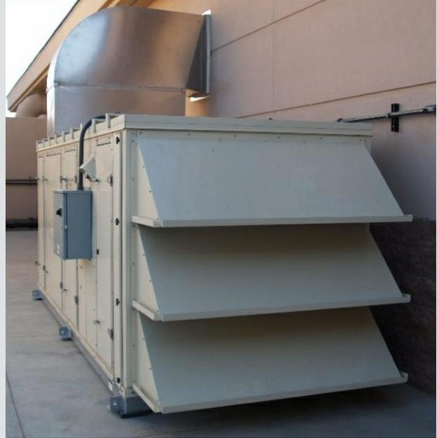
Supply Air Handler with Ionizer Section
