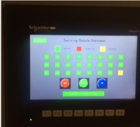
*the **negative 32°C minimum design temperature** through inclusion and control of module thermostats, motorized thermal dampers, and hydronic heaters. Integration with the facility SCADA system will provide real-time status of the ion generators and other important module components."*
